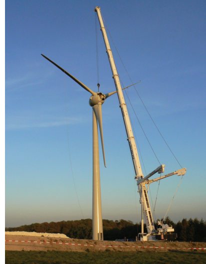
Wind Turbine Construction
